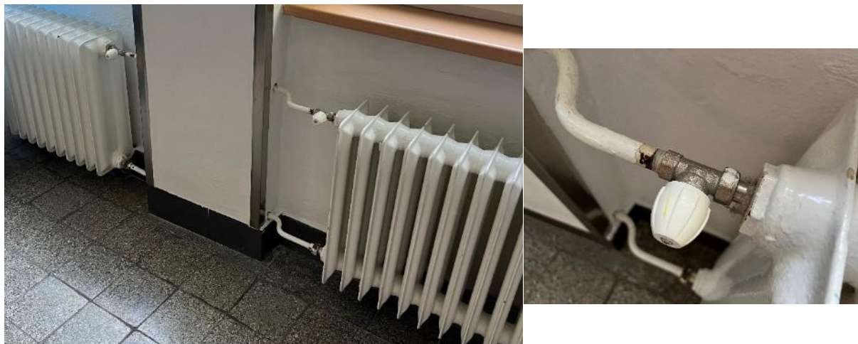
Obr. Detail OT a ventilu
