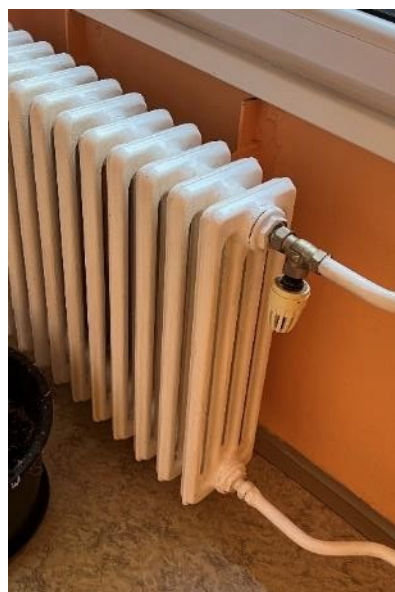
Obr. Detail OT s TRV
