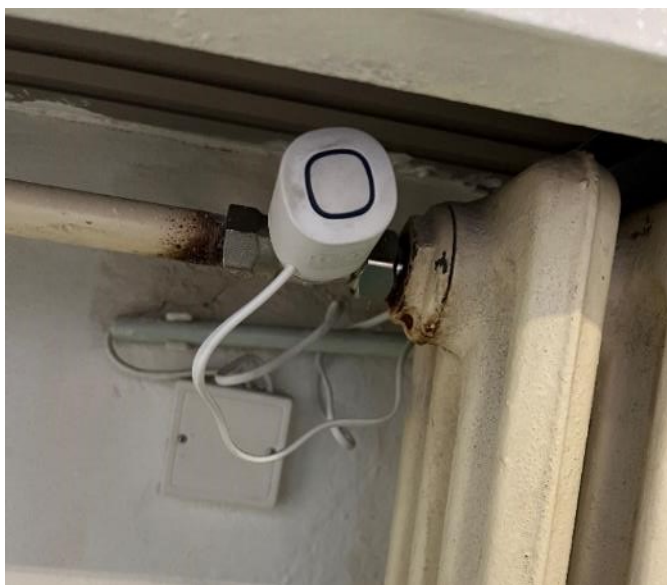
Obr. Detail IRC hlavice
