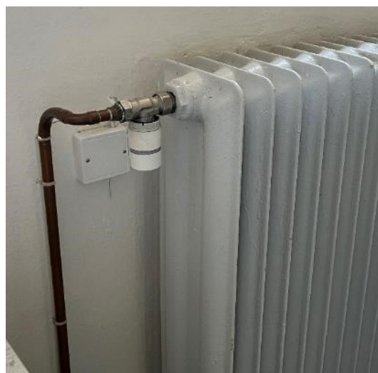
Obr. Detail OT v kabinetu – IRC hlavice
